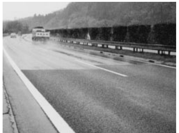
Fig.5 Pavement with better drainage, which is designed to maintain traction and prevent water splashing up from the road's surface
