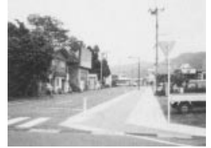
Fig.4 Space for cyclists in Futatsuimachi, Akita Prefecture (Bicycle passing zone is physically separated.)
